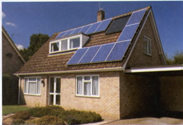
Solar panels on the roof help provide heat and electricity.
